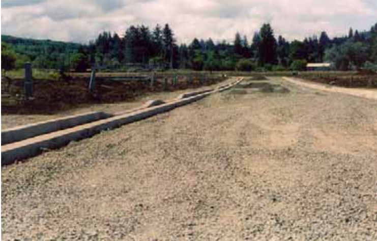
Oak Flats Under Construction
